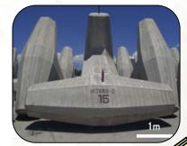
Wave-dissipating blocks with uneven surface
